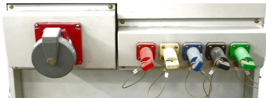
Figure 2.4- Additional Power Supply
